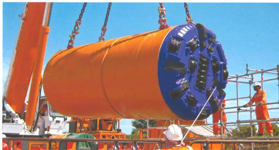
Construction of sewerage system by pipe jacking technology is the most advantage success. Process will include the following steps:
